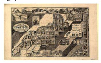
Ultimately, the Comstock mines went thousands of feet deep (over 1000 meters) involving intricate underground wooden structures to shore up the loose soil.
